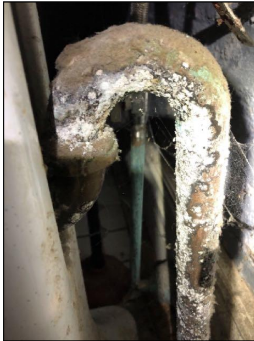
Corroded drain pipe
