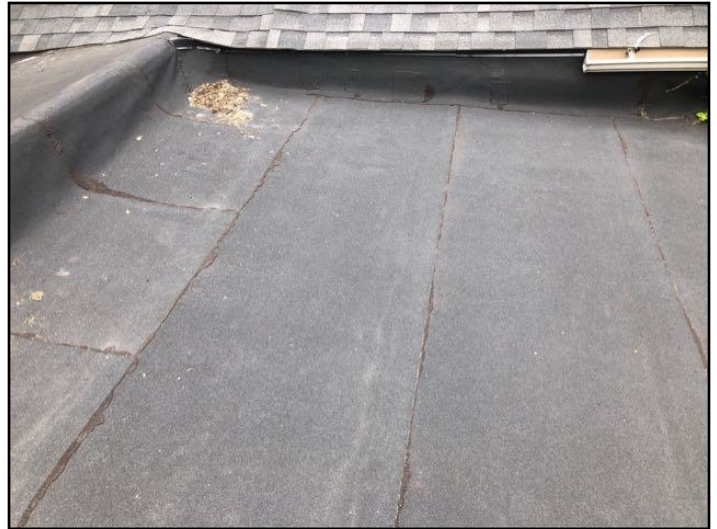
Modified bitumen membrane
