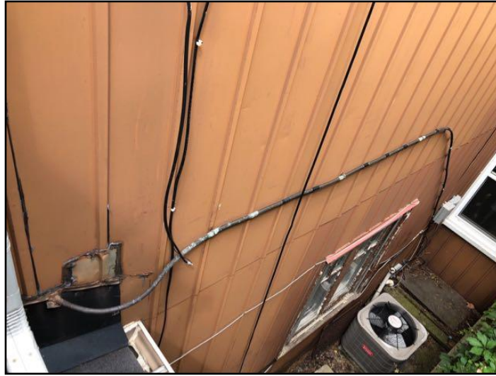
Copper tubing not properly labeled
