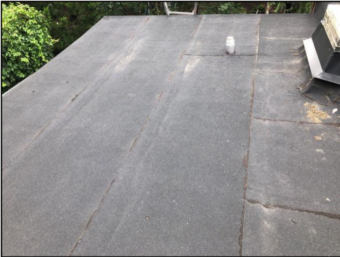
Modified bitumen membrane
