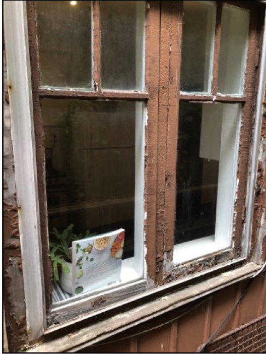
Paint and caulking - deteriorated / missing
