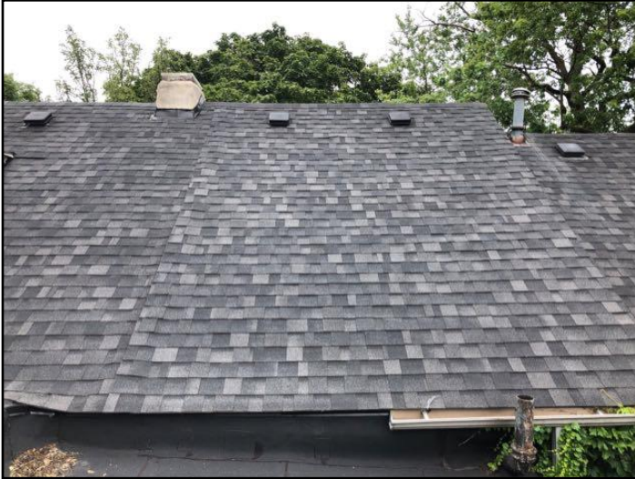
Asphalt shingles
