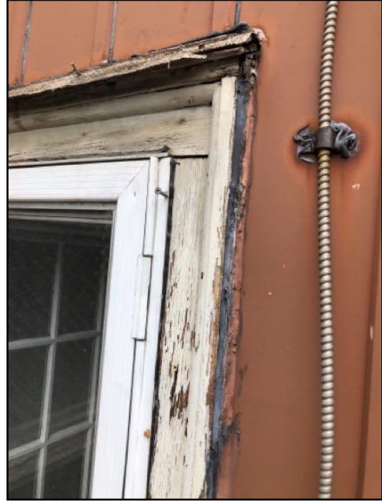
Paint and caulking - deteriorated / missing
