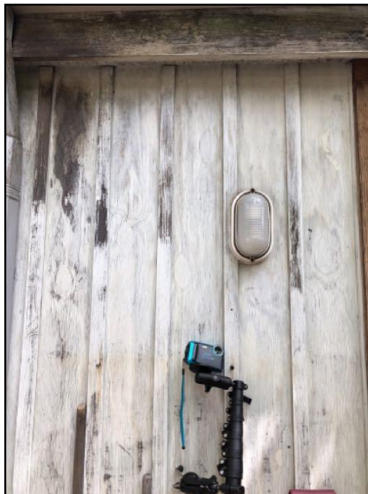
Paint or stain - needed
