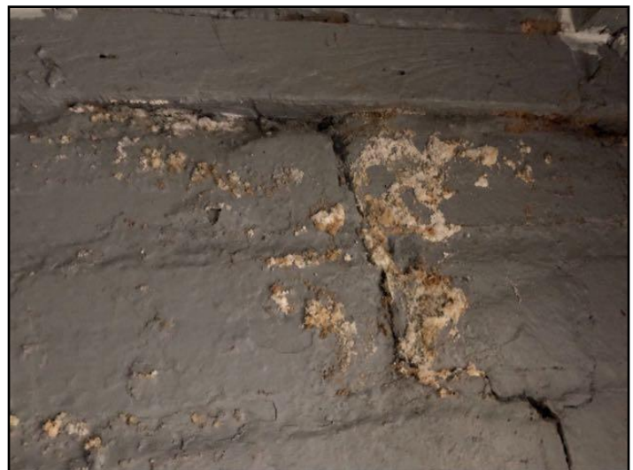
Efflorescence
