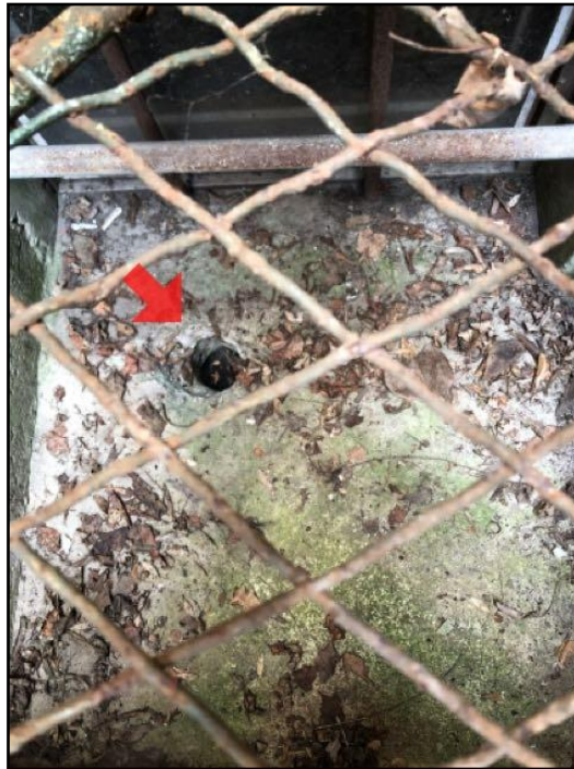
open drain at window well
