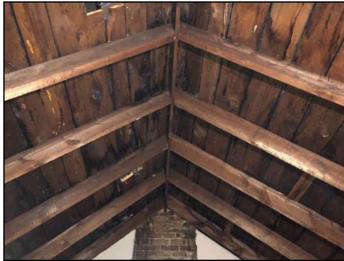
Missing collar ties
