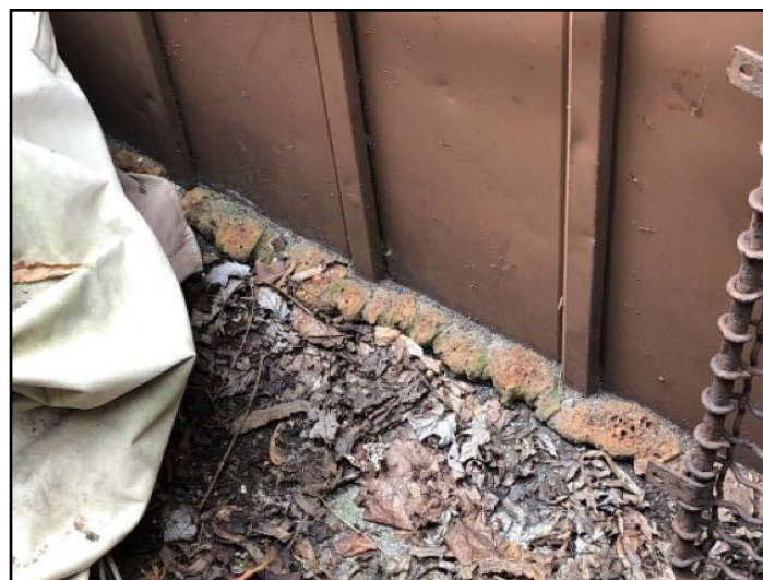
Too close to grade
