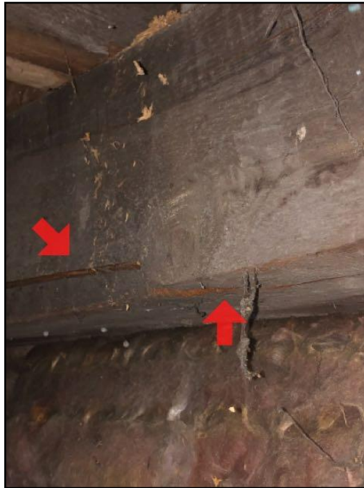
cracked beam
