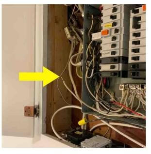
7.5.3 **100** amp service. breaker panel with some room for expansion. No significant visible defects inside the panel.
