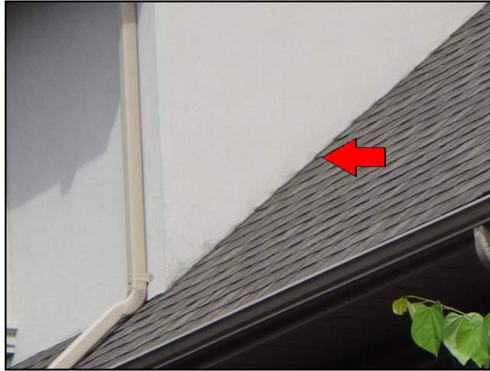
Clearance to siding inadequate
