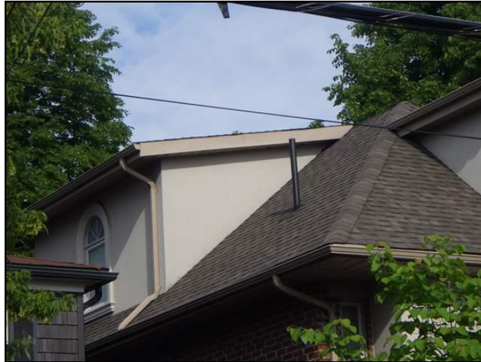
Asphalt shingles
