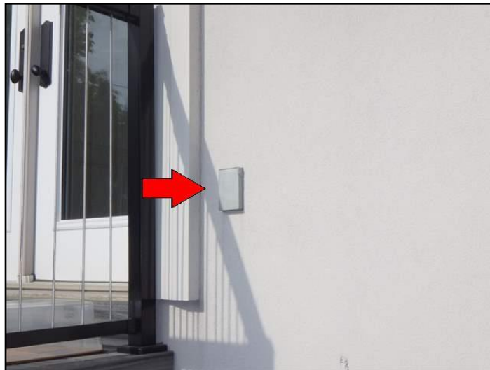
Test faulty on GFCI/GFI (Ground Fault...
