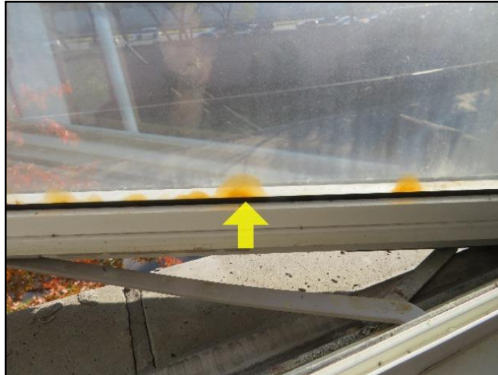
Lost seal on double or triple glazing
