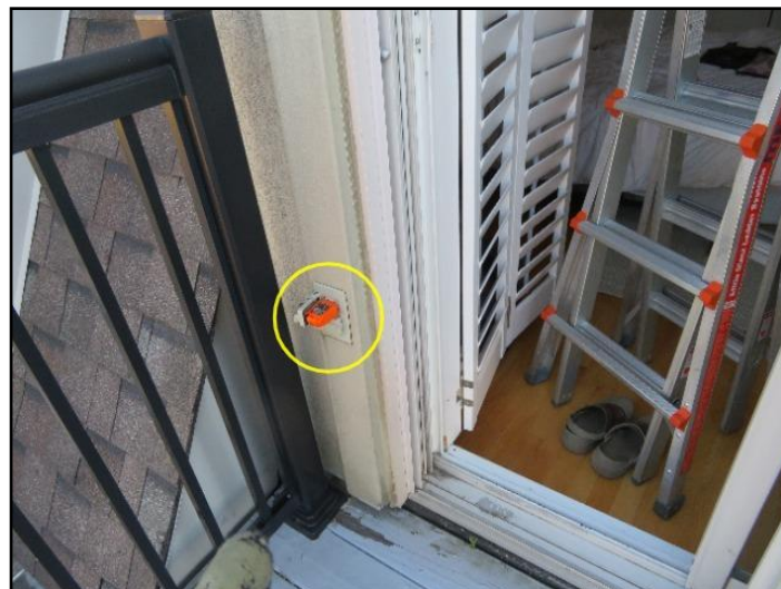
No GFCI/GFI (Ground Fault Circuit...
