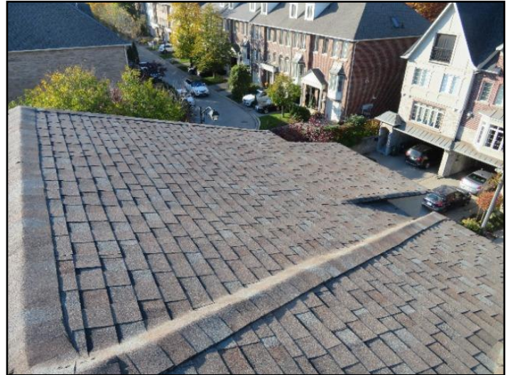
Asphalt shingles
