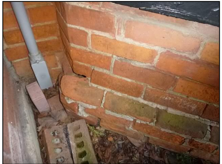
Mortar deterioration, a few damaged bricks
