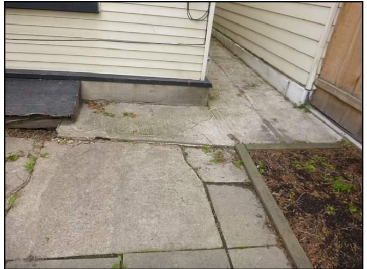
Improper slope or drainage- rear
