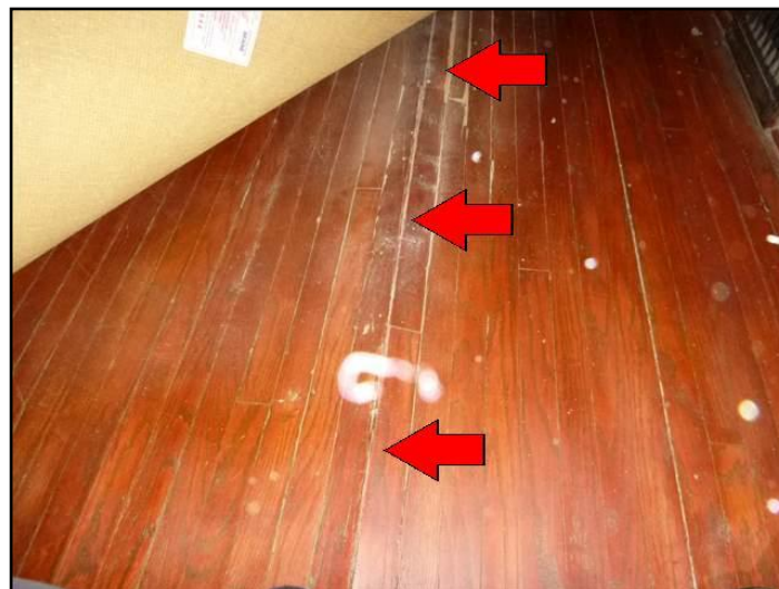
Damage (buckled flooring)
