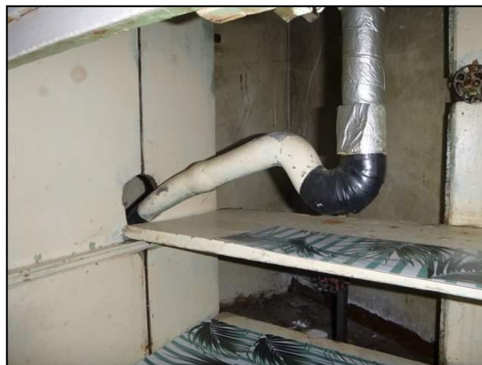
Lead drain piping at kitchen sink (typ.)
