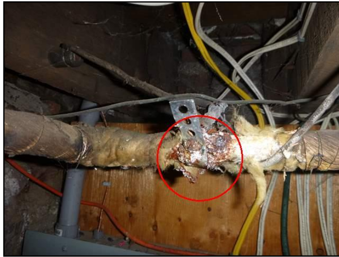
Leak at pipe support
