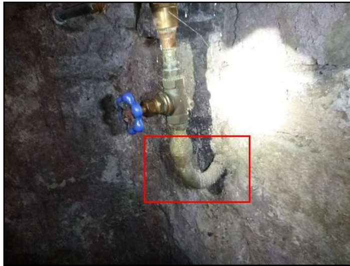
Lead supply pipe from utility
