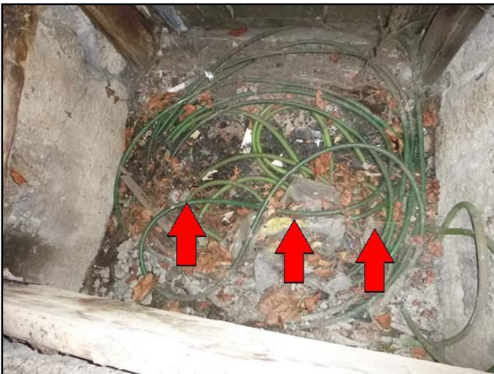
no drain visible, window close to grade level
