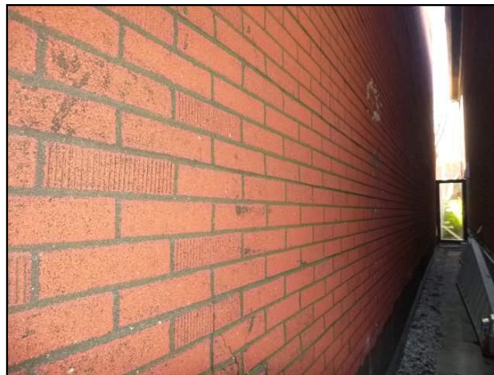
Insulbrick cladding at side wall
