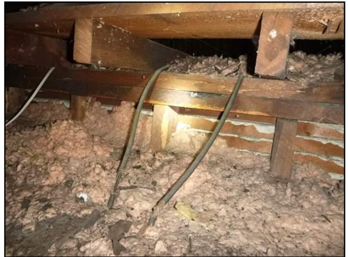
Remnants of knob-and-tube (not energized)
