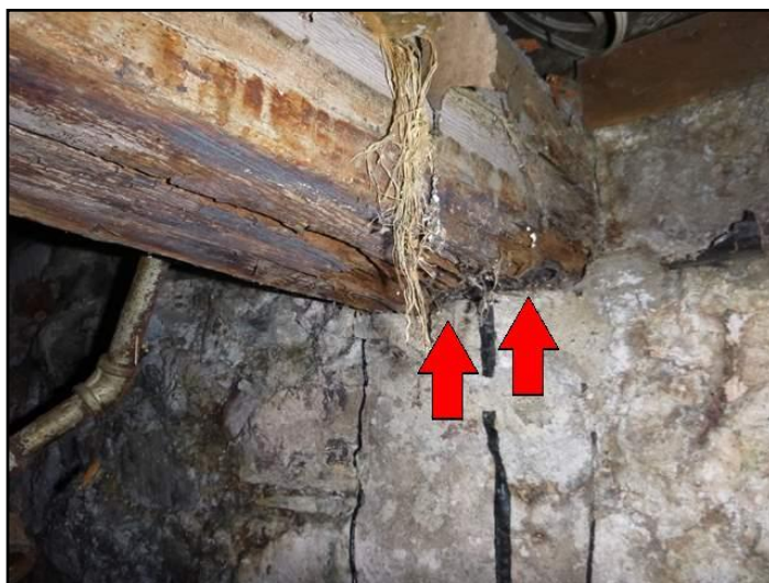
Damage at beam end
