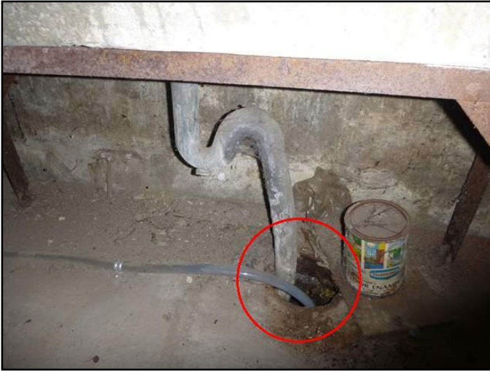
Tub drain discharges to floor drain?
