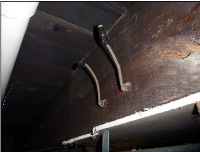
Remnants of knob-and-tube (not energized)
