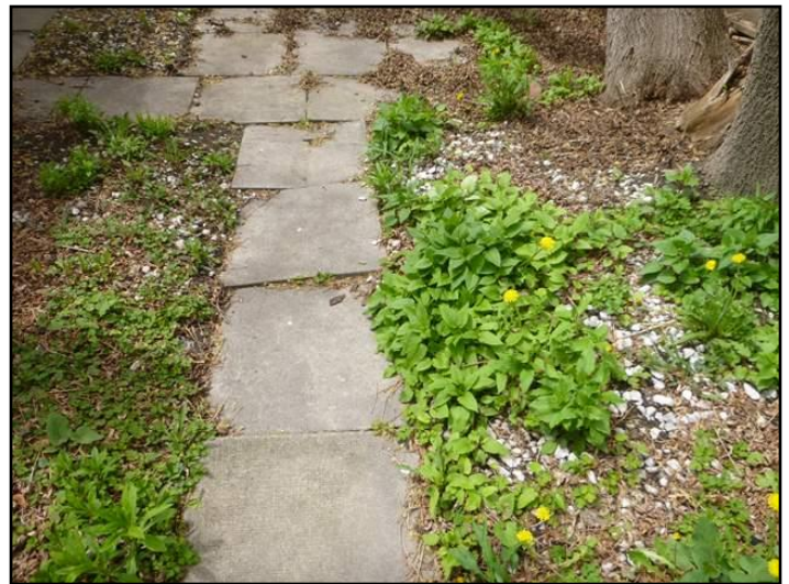
Uneven (trip hazard)- rear
