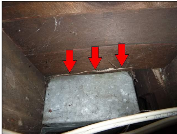
Insulation material at register not determined
