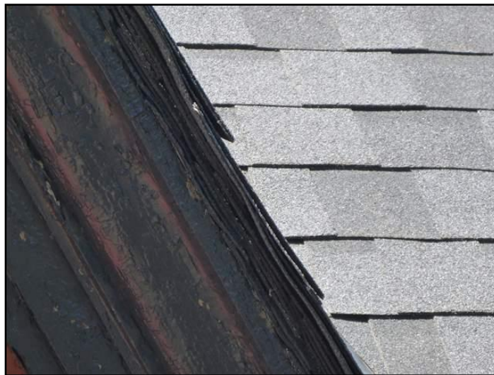
Multiple layers of shingles noted
