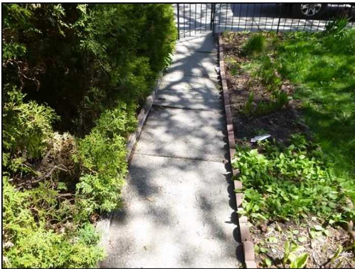
Uneven (trip hazard)- front
