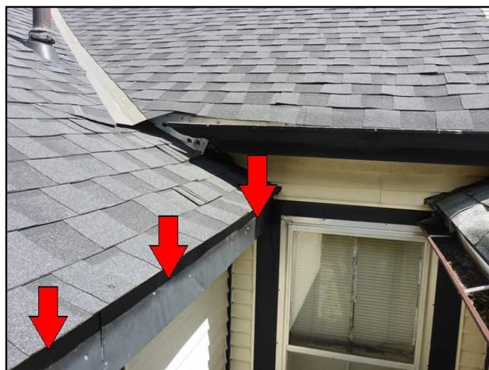
Missing gutters and downspouts
