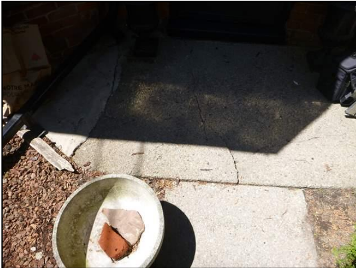
Improper slope or drainage- front
