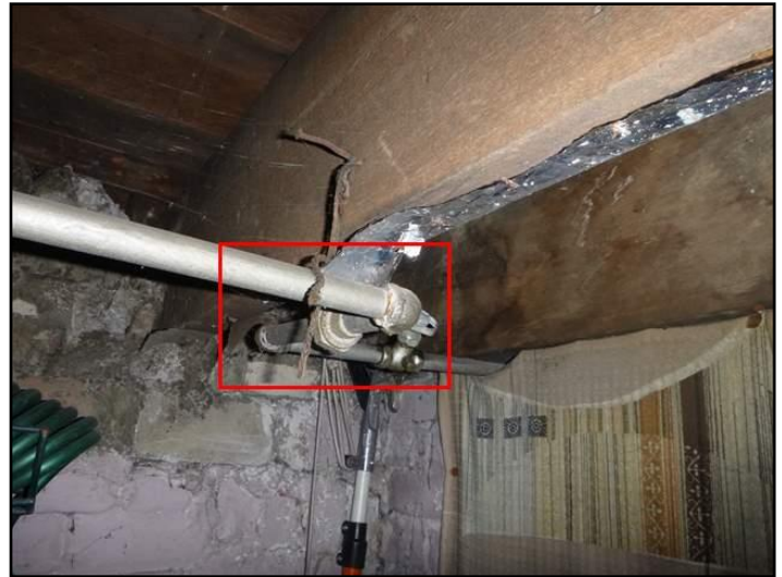
Galvanized steel supply piping noted
