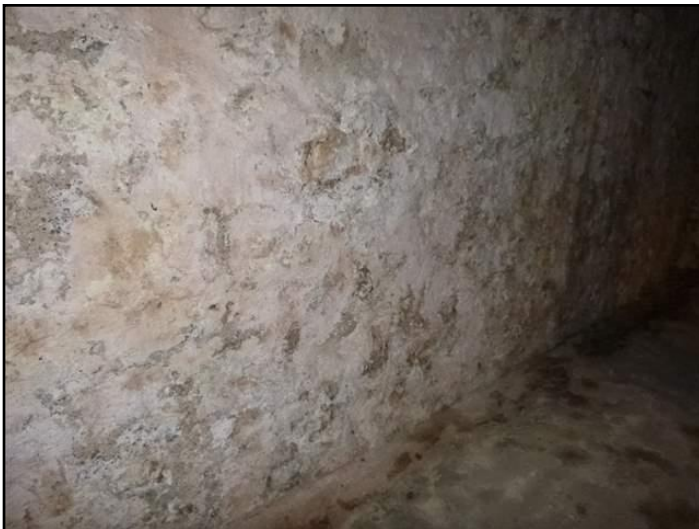
Efflorescence
