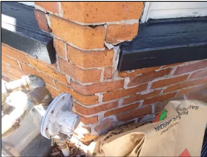
Mortar deterioration, loose bricks
