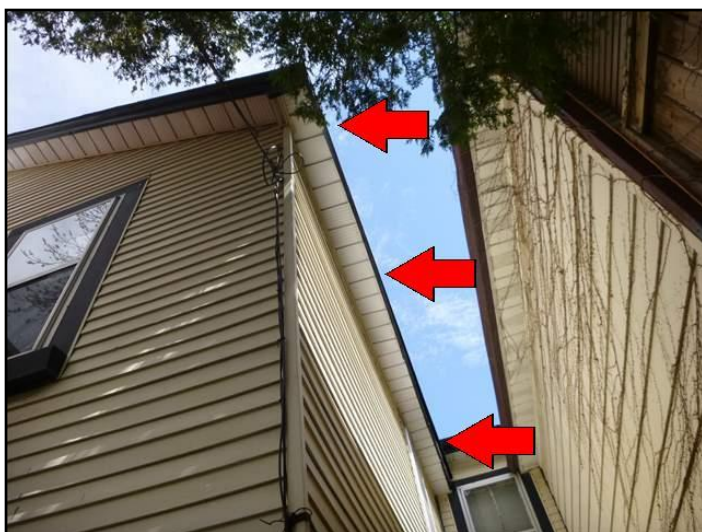
Missing Gutters and downspouts
