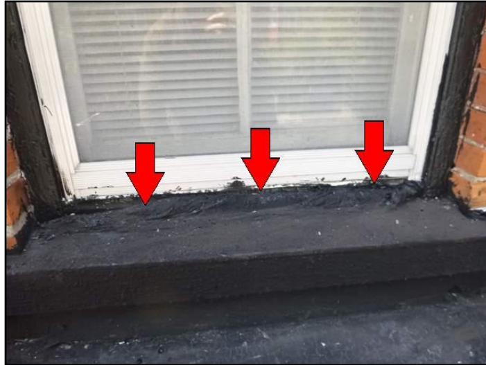
Damage- temporary repair noted
