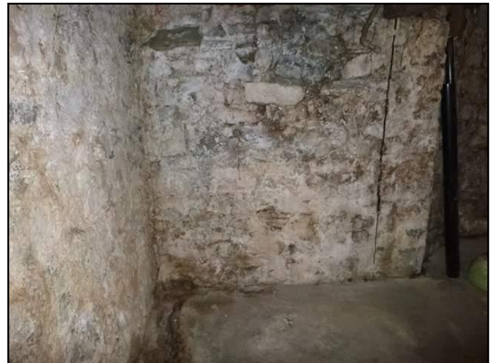
Efflorescence
