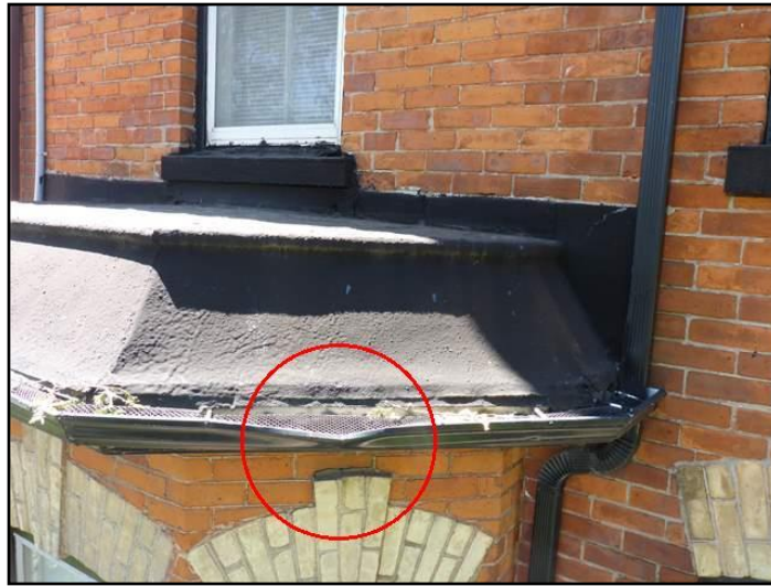
Damaged gutter at front bay
