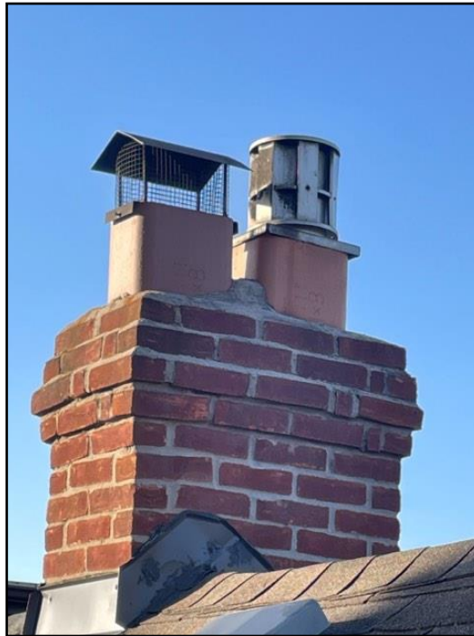
Missing chimney cap
