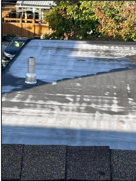
Modified bitumen membrane
