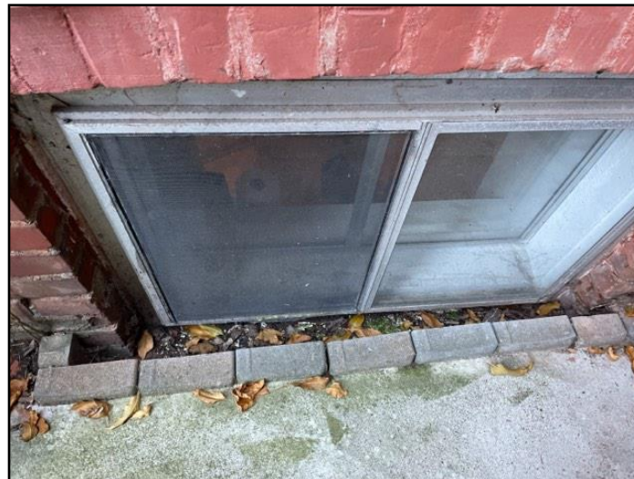
Window close to grade in well
