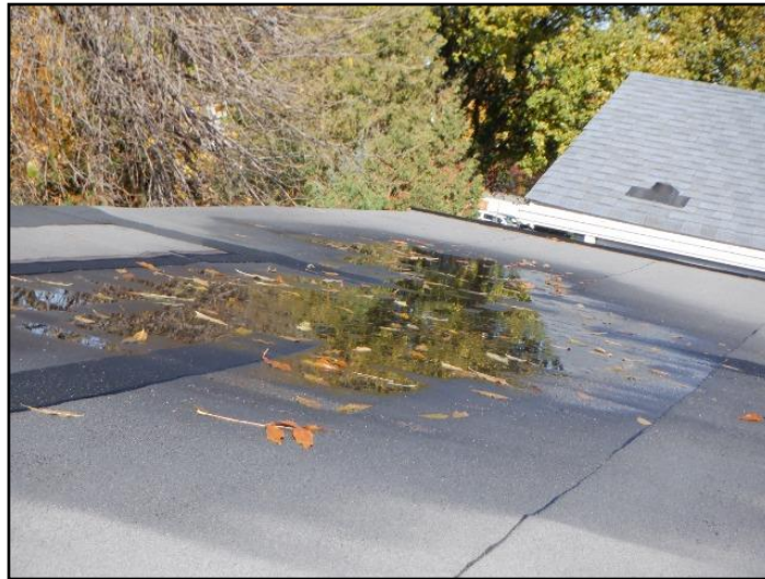
Water ponding on the roof
