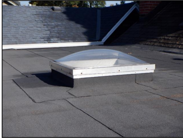
Skylight(s) - vulnerable area for leaks.
