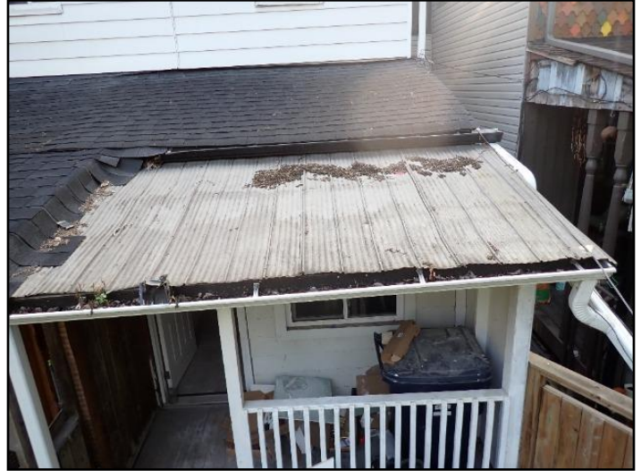
Rear porch awning
