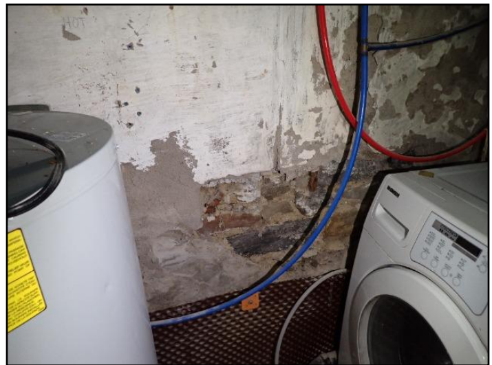
Ex. laundry area
