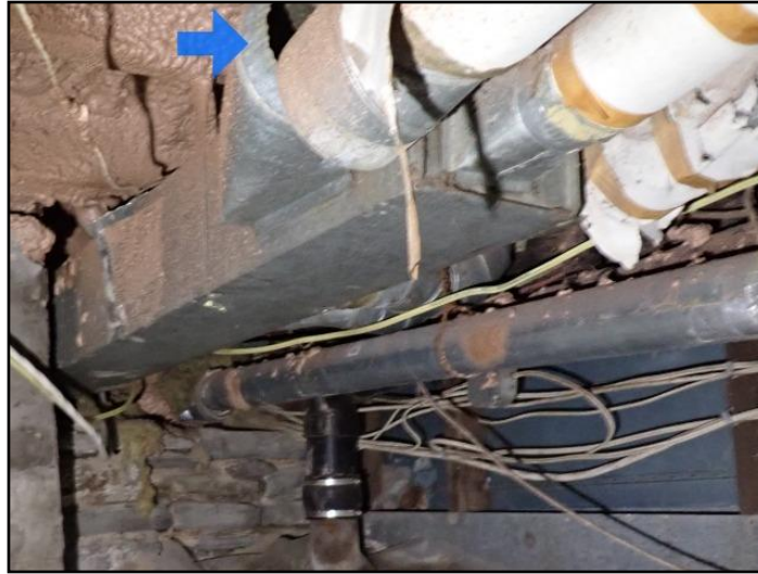
Disconnected ducts
