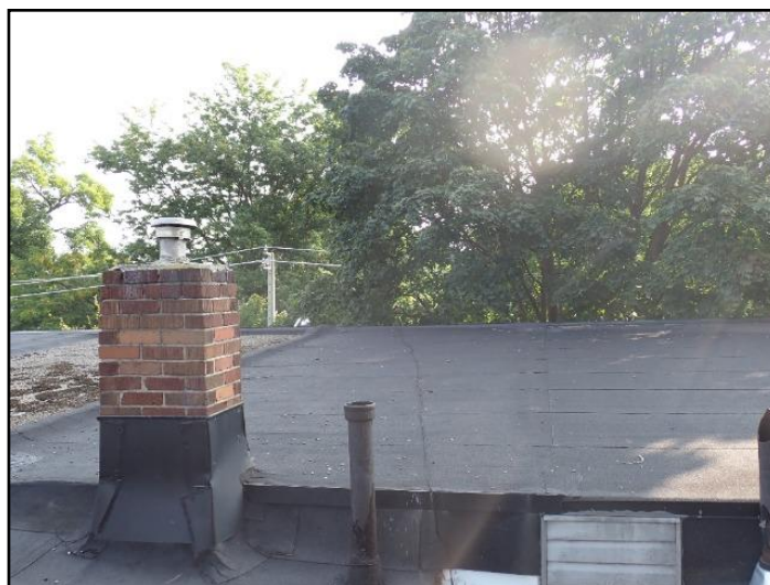
Main roof rear
