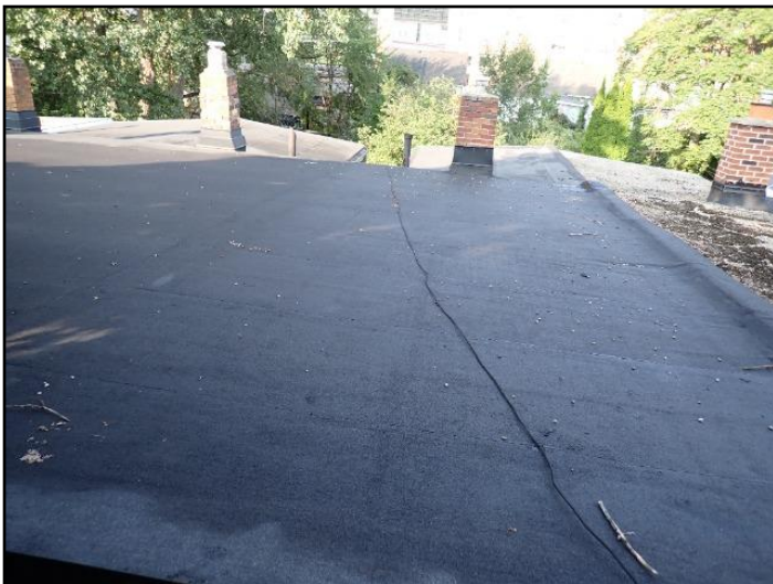
Main roof front
