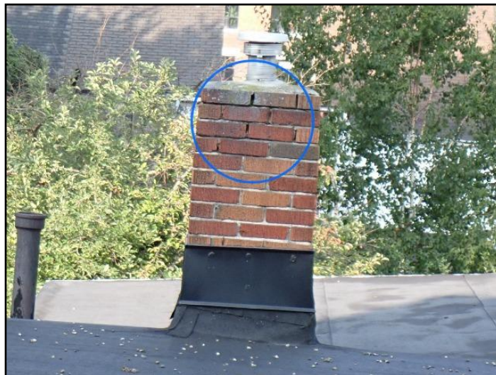
Deteriorated mortar
