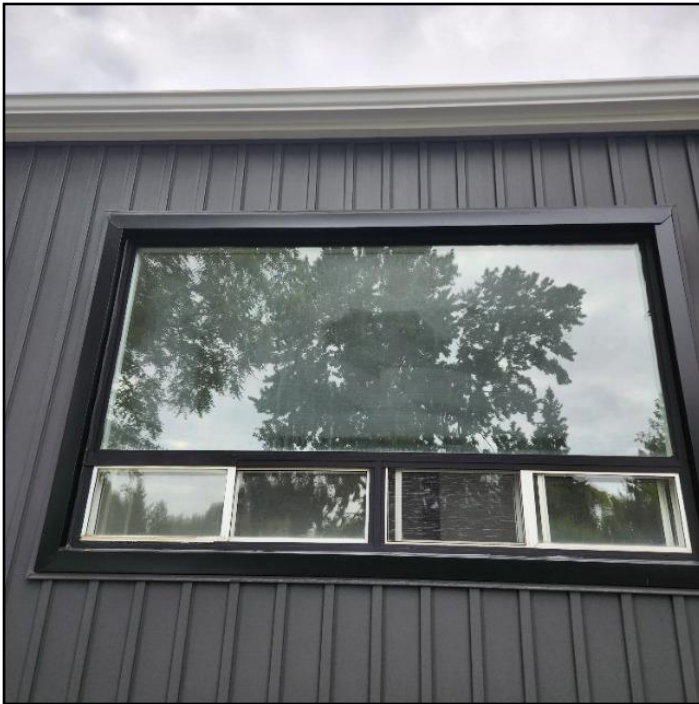
28. Lost seal (Exterior View)
