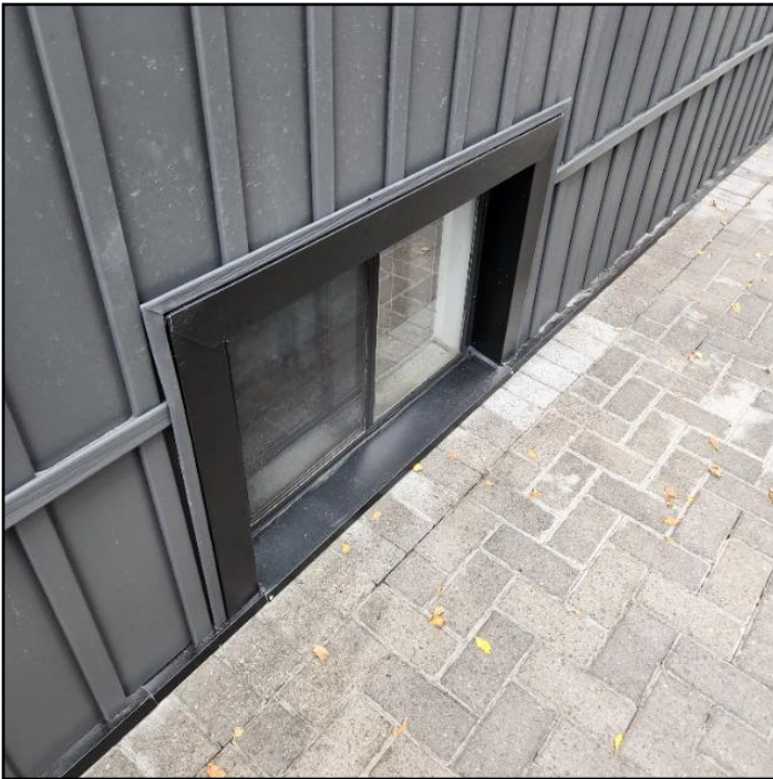
3. No window well installed
