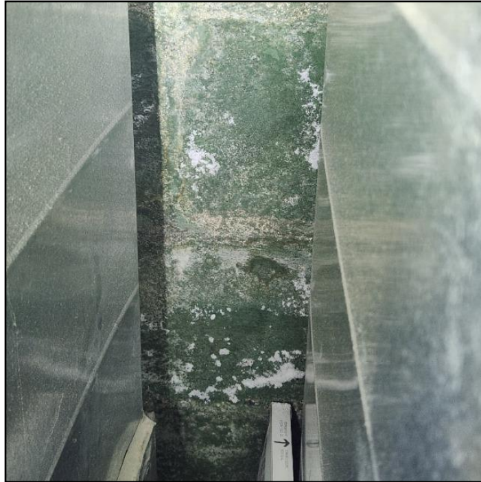
33. Efflorescence
