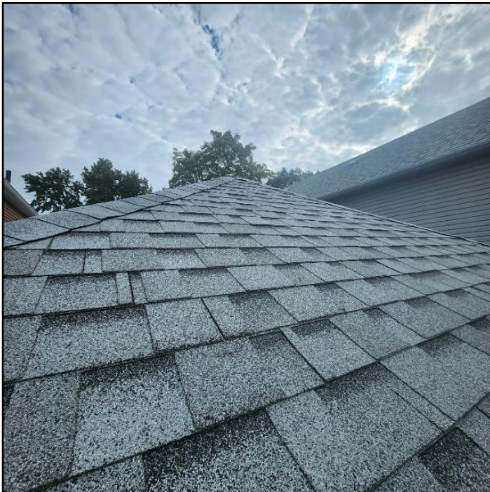
1. Asphalt shingles
