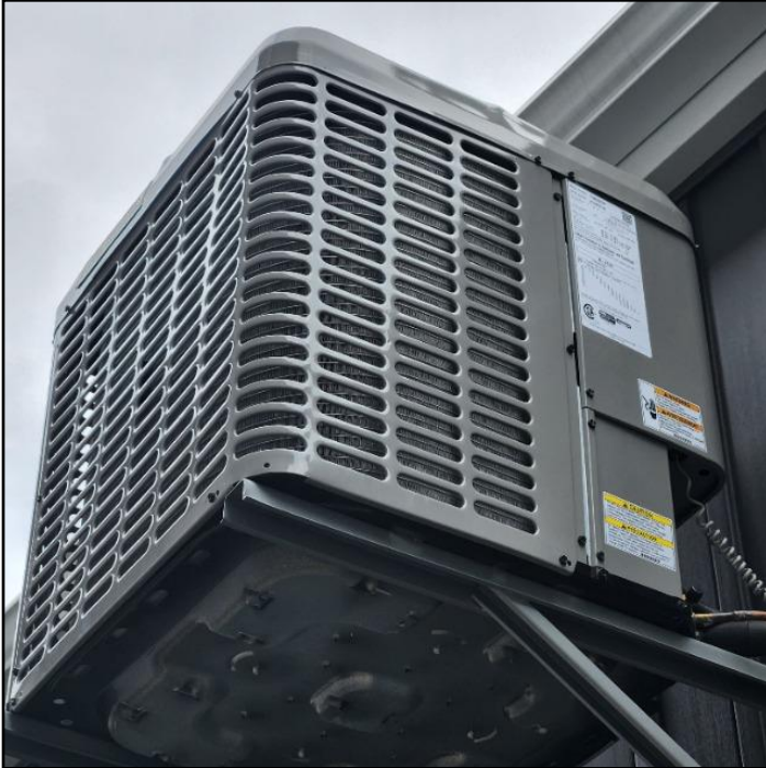
14. Air cooled Condenser
