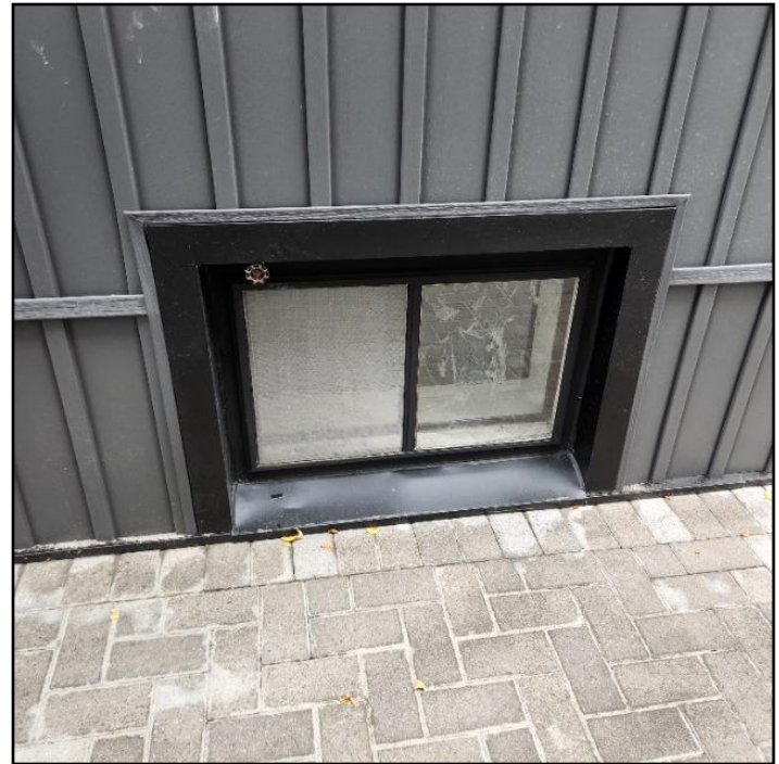
4. No window well installed
