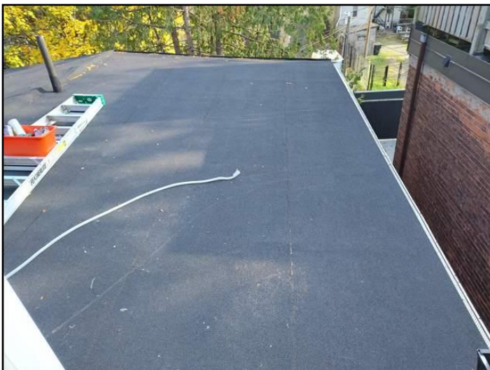
Modified bitumen membrane
