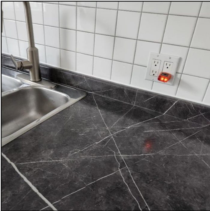
12. upgrade plug to GFCI
