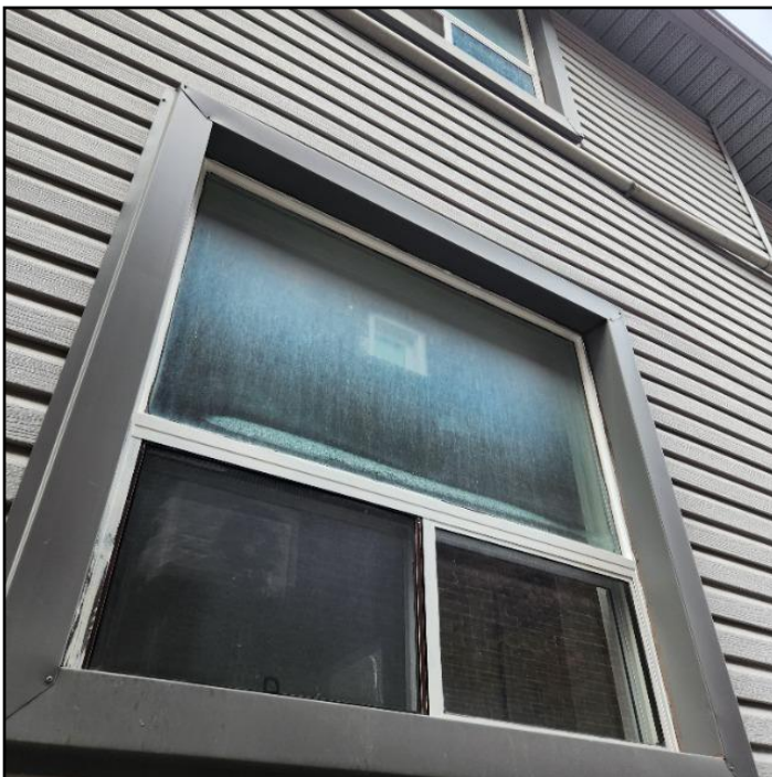
33. Lost seal on double glazing
