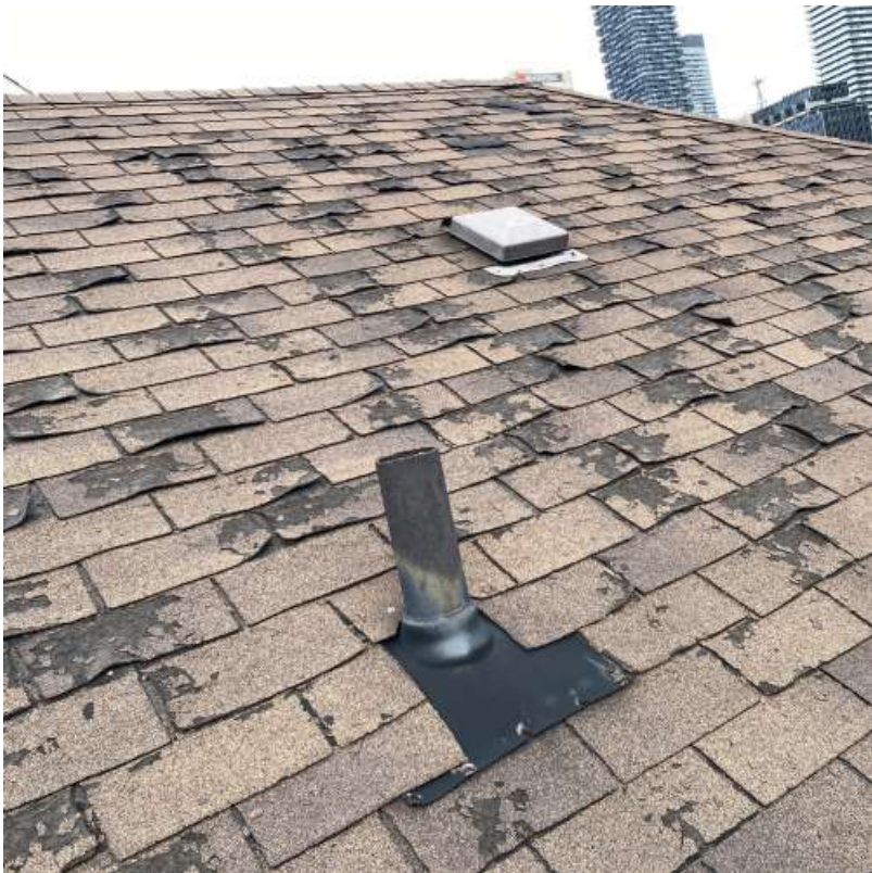
A view of the south face of the main roof.
