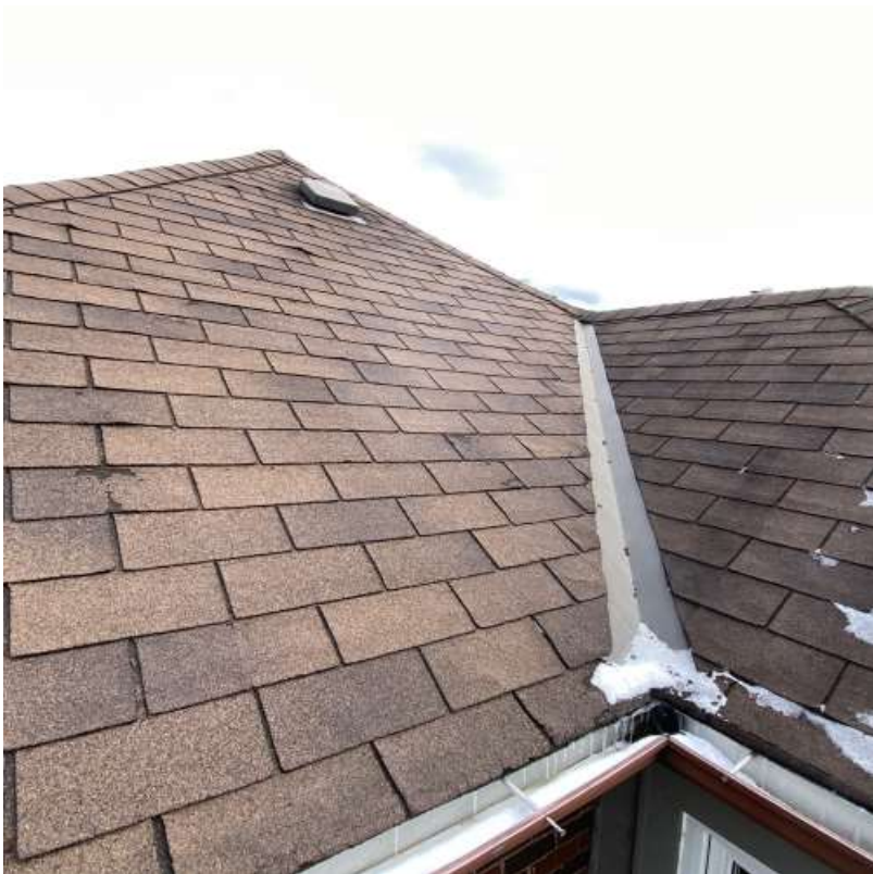
A view of the west face of the main roof.
