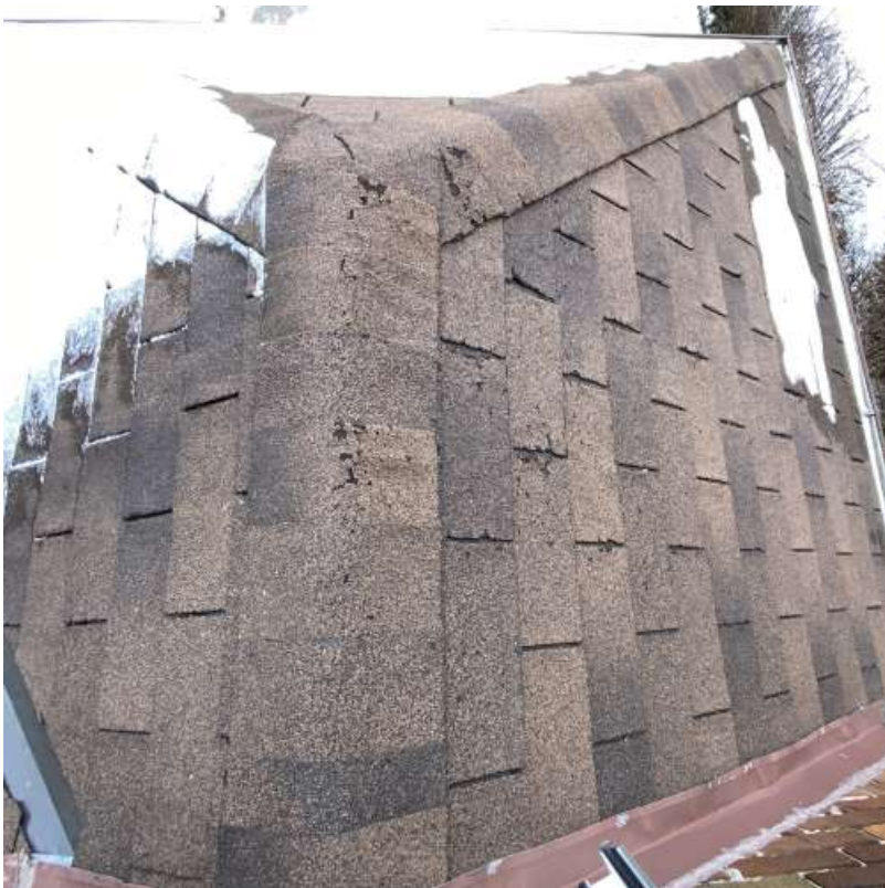
A view of the roof coverings at the front overhang roof.
