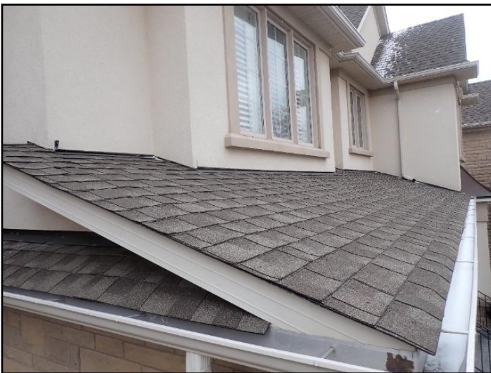
Shingles are in good/aging condition
