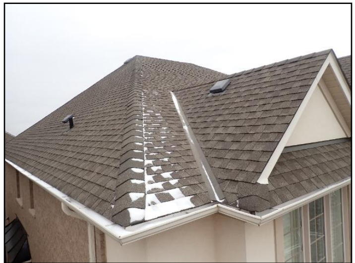
Shingles are in good/aging condition
