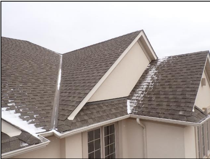
Shingles are in good/aging condition
