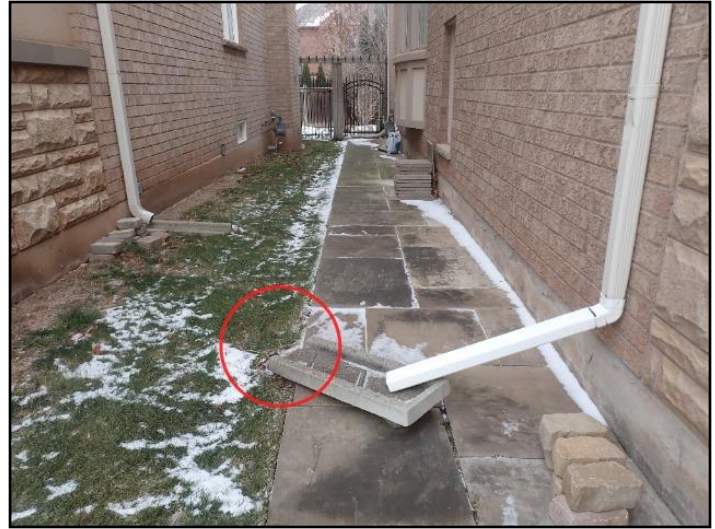
Maintain discharge well away from foundation
