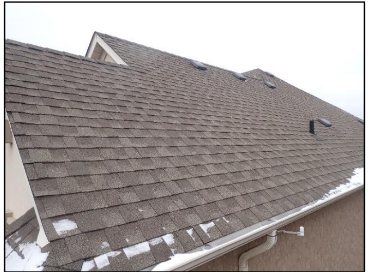
Shingles are in good/aging condition
