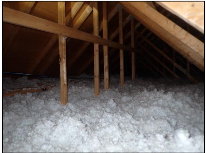
Insulation is evenly distributed
