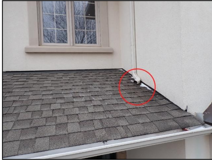
Discharge onto roofs
