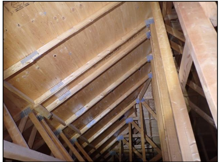
Roof sheathing is clean
