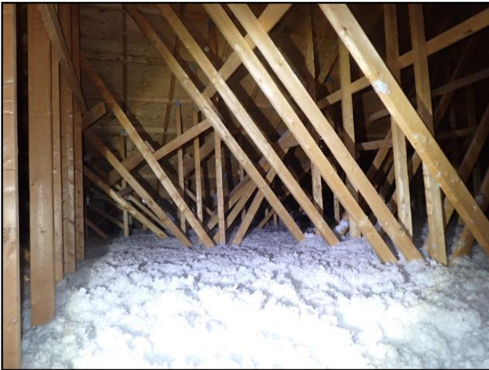
Insulation is evenly distributed
