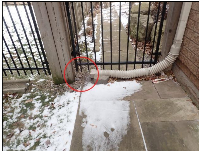
Maintain discharge well away from foundation
