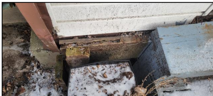
36. Rot or insect damage
