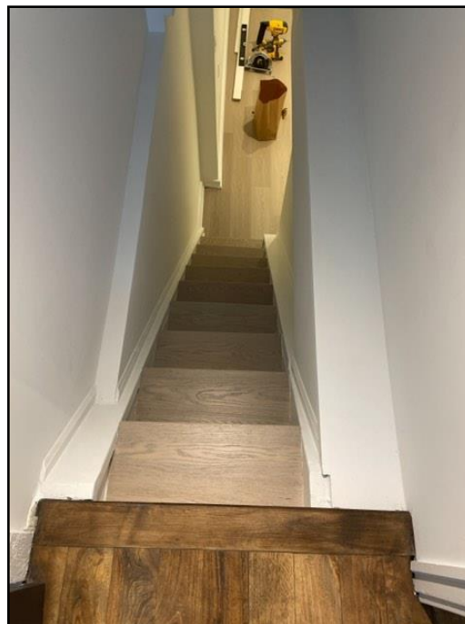
Missing handrail
