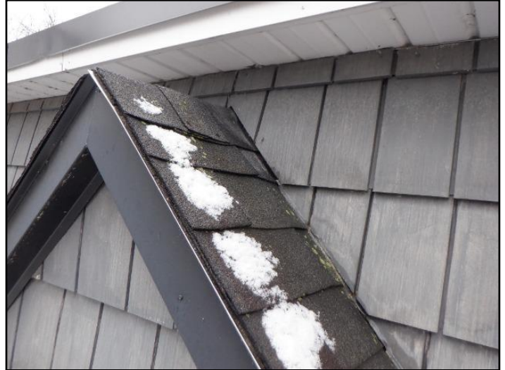
Asphalt shingles
