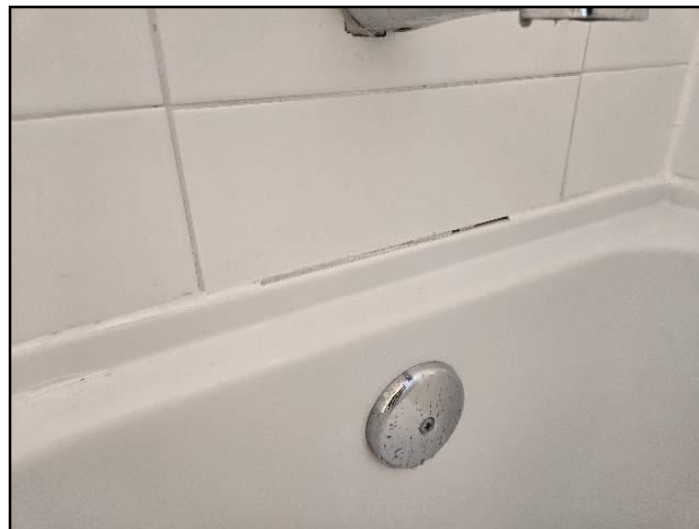
Caulking loose, missing or deteriorated
