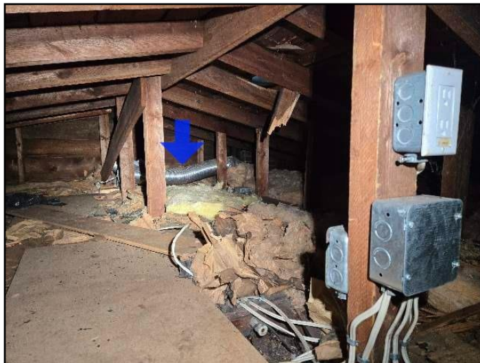
Not insulated in unconditioned space
