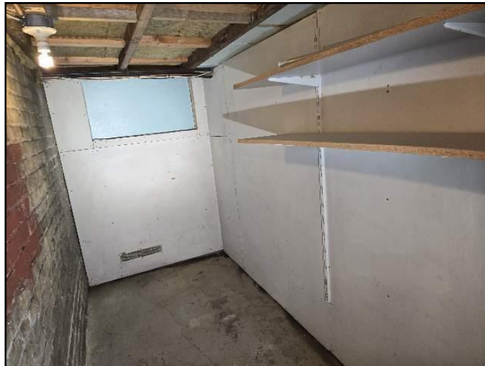
Finished risk of condensation problems
