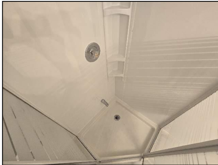
Caulking loose, missing or deteriorated
