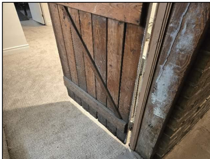
Door should be insulated
