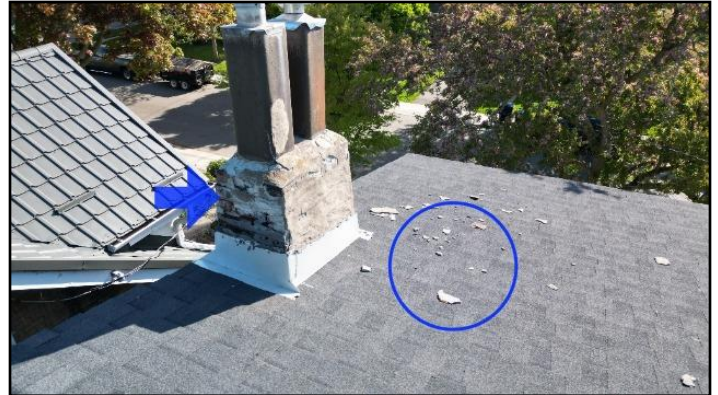
Ex. Chimney - Parging damaged
