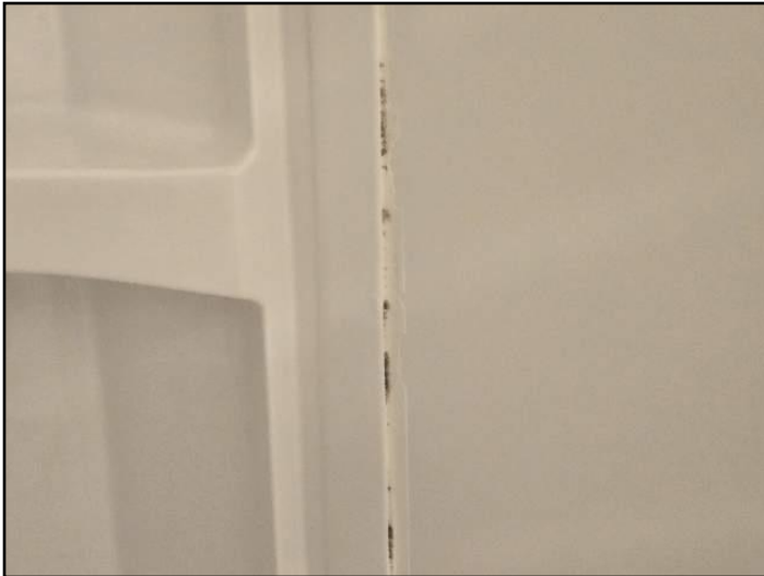
Caulking loose, missing or deteriorated
