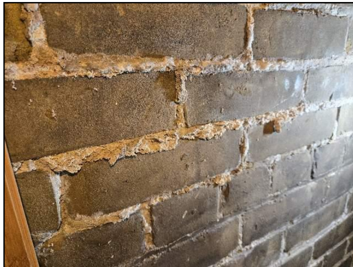
Efflorescence
