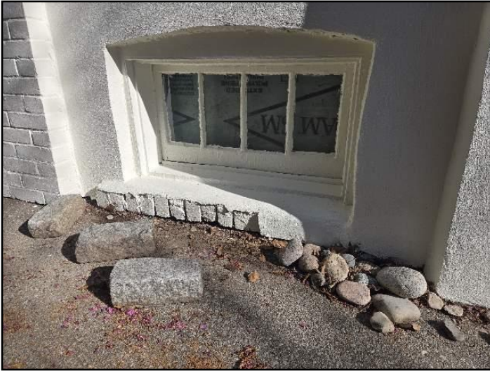
Ex. Left side - Parging missing
