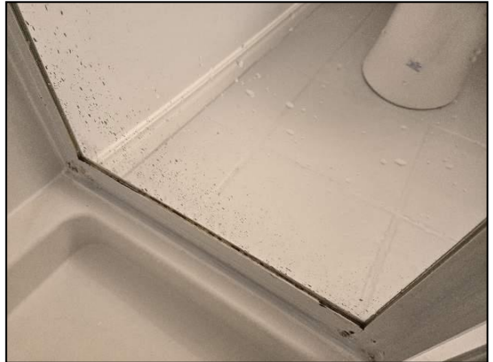
Caulking loose, missing or deteriorated
