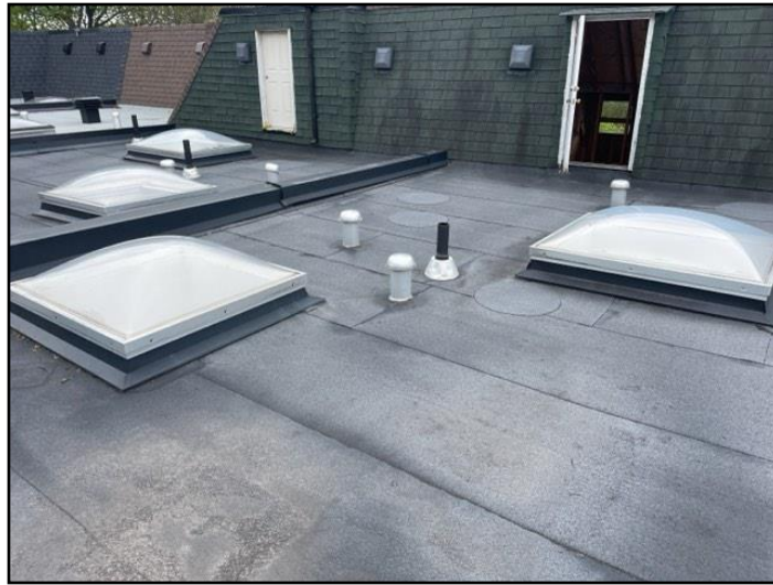
Skylight(s) - vulnerable area for leaks.
