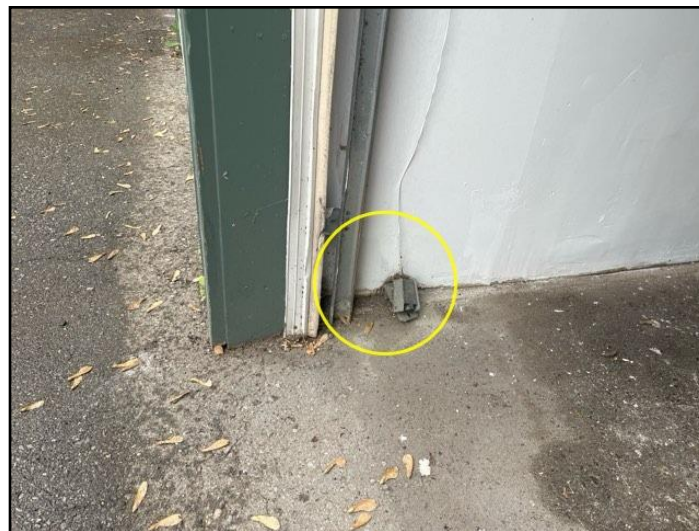
Example: Sensors damaged
