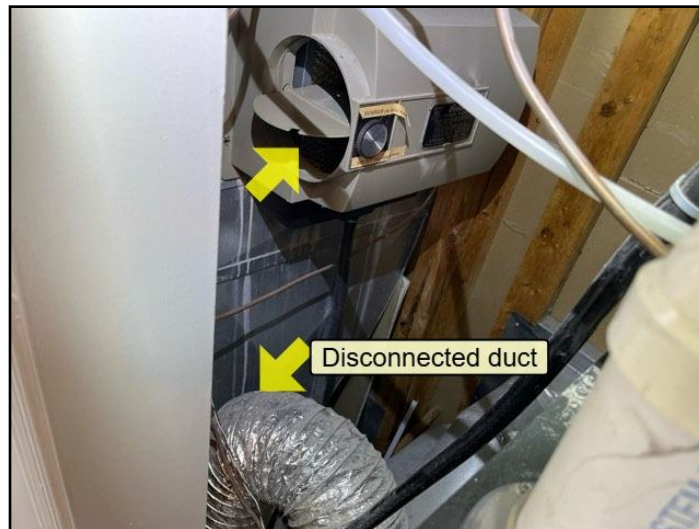
Ductwork damage
