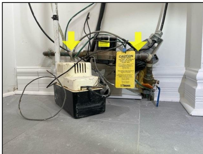
No jumper for meters and valves
