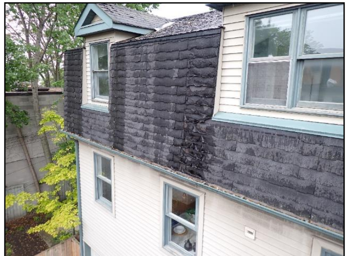
Front, Lower (siding): At end of life
