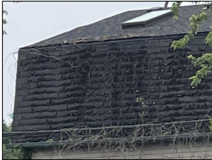
Rear, Lower (siding): At end of life
