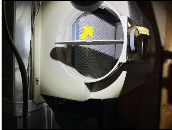
Clogged pad, mesh or nozzle
