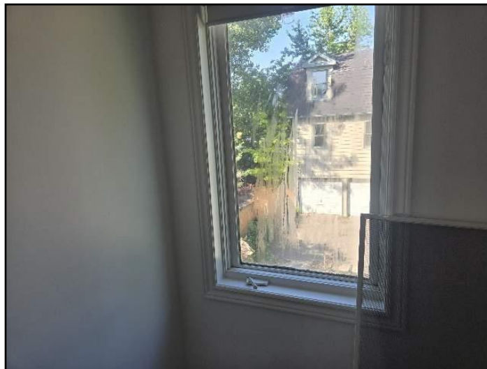
Lost seal on double or triple glazing
