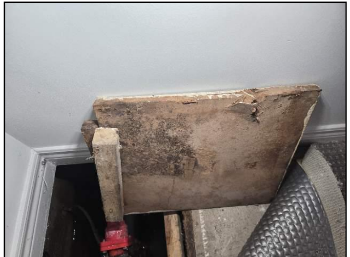
Cover swollen and delaminating
