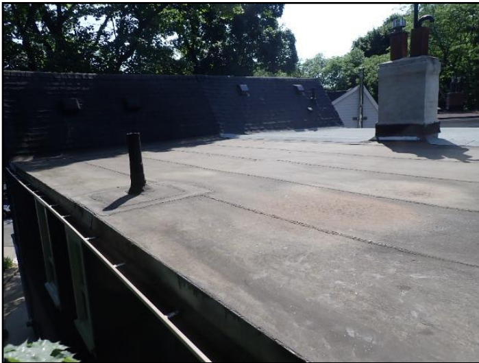
Modified bitumen membrane
