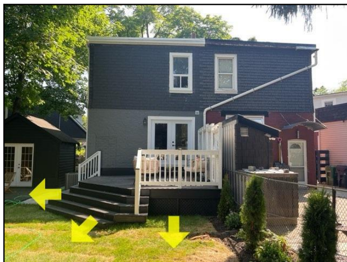
Improve grading as necessary
