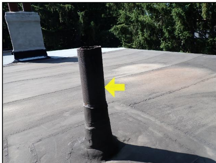
Cast iron waste stack
