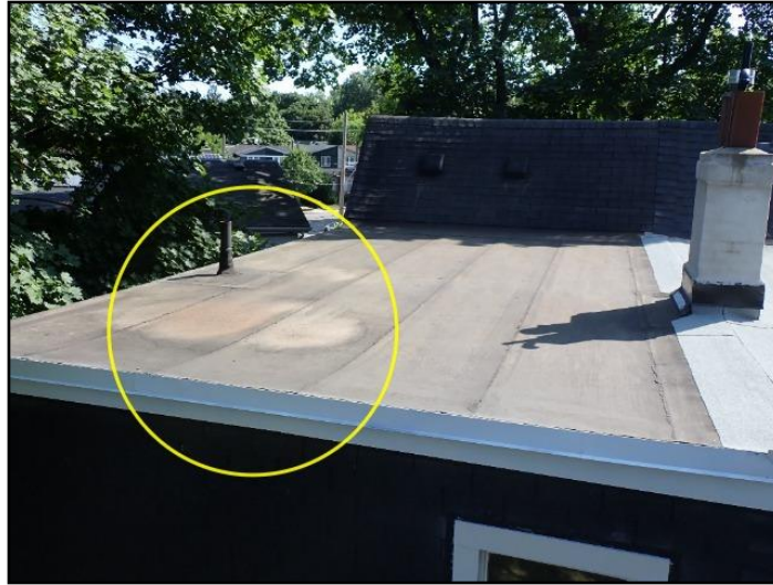
Water ponding on the roof
