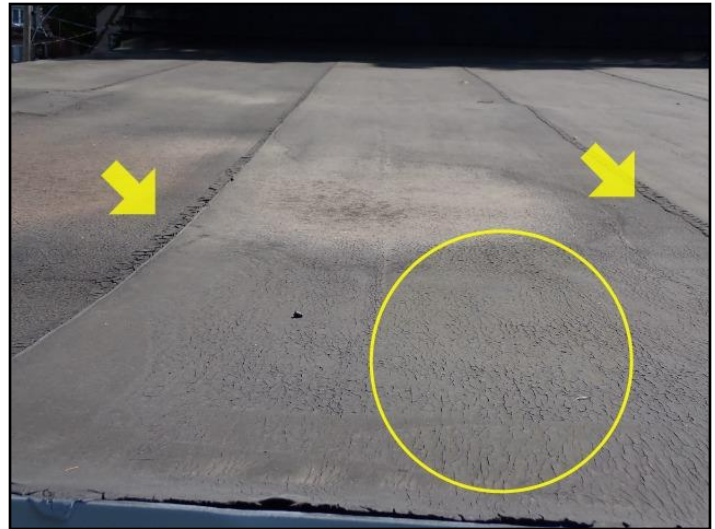
Seams degrading, Alligatoring surface
