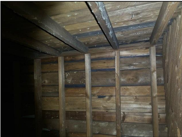
Sloped Roof: Plank sheathing / Rafters
