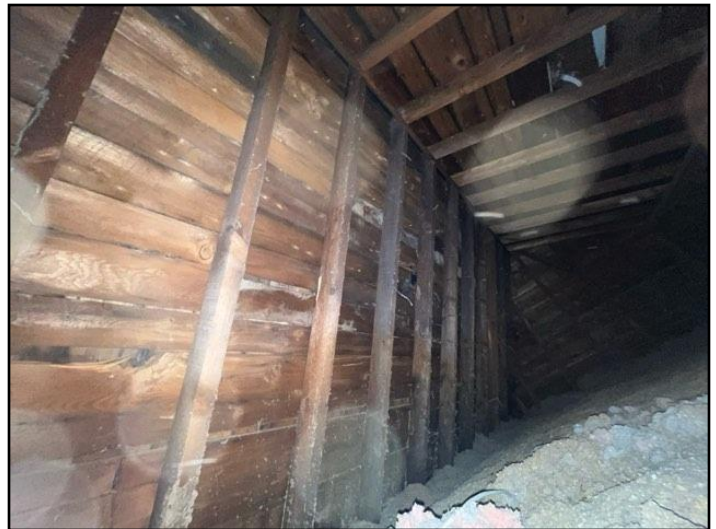
Sloped Roof: Plank sheathing / Rafters
