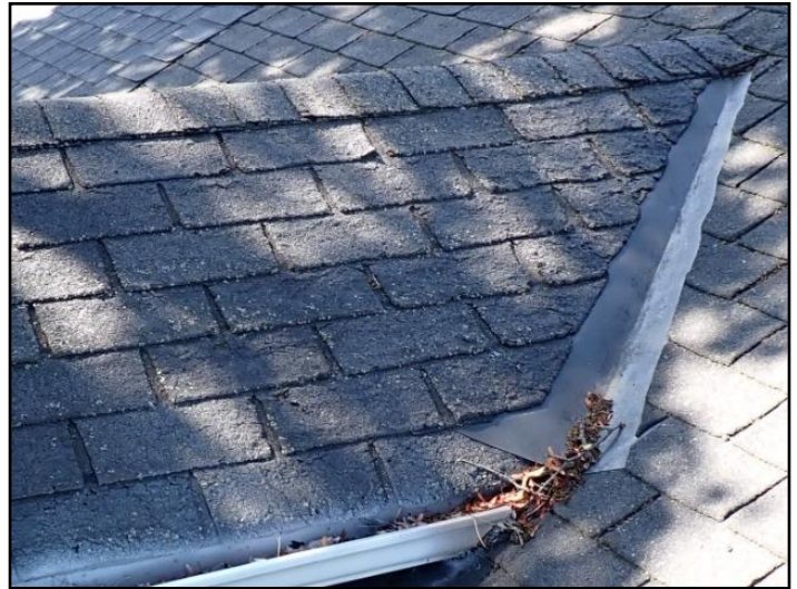
Cupping, Curling, Broken edges
