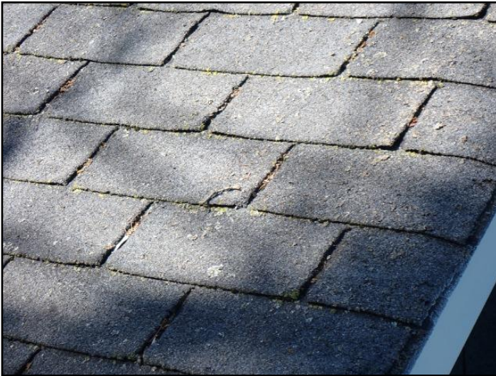
Loss of granular material, widening slots
