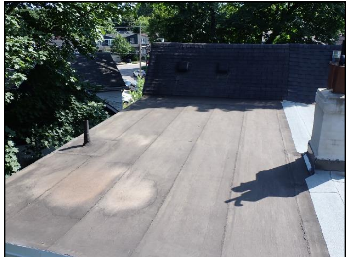
Modified bitumen membrane
