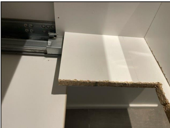
Doors or drawers missing or loose
