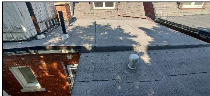
Modified bitumen membrane
