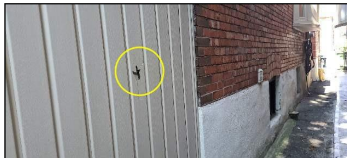
Damaged siding
