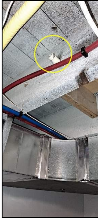
Remnants of knob-and-tube wiring noted
