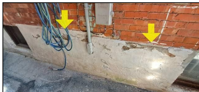
Parging damaged
