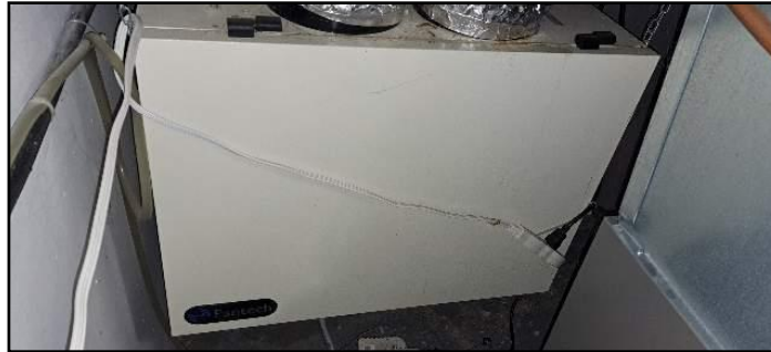
Heat recovery ventilator (HRV)
