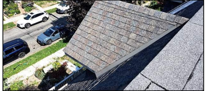
Asphalt shingles
