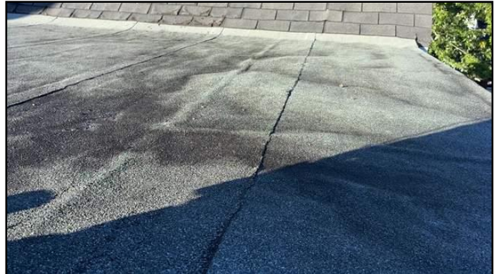
Modified bitumen membrane
