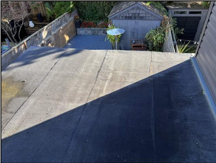
Modified bitumen membrane
