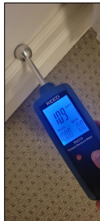
81. Moisture meter results
