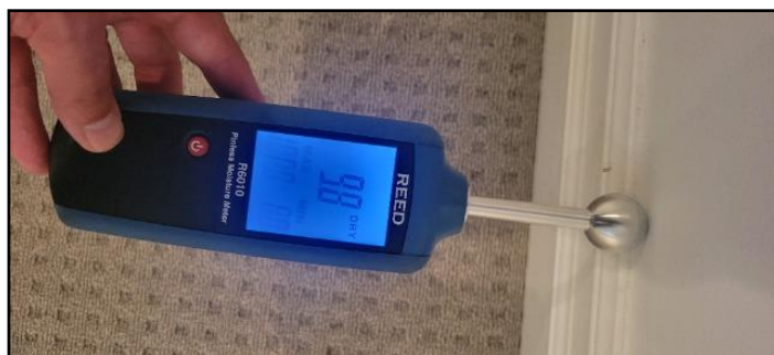
86. Moisture meter results
