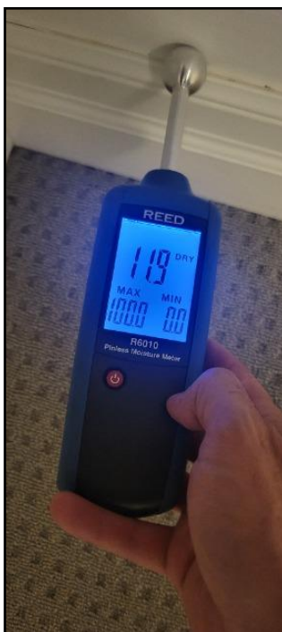
80. Moisture meter results
