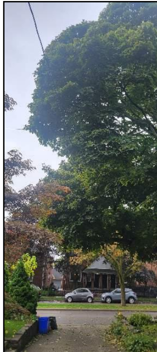
46. Branches / vines interfering with wires
