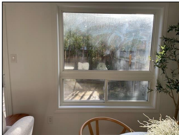
main floor rear window
