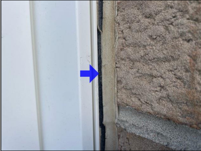
Caulking deteriorated
