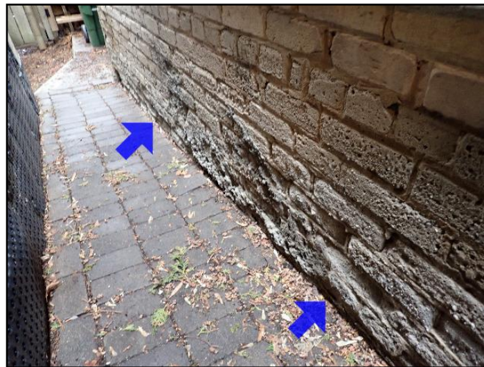
Masonry deterioration
