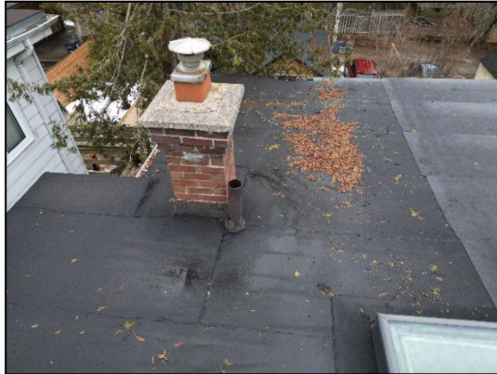
Modified bitumen membrane
