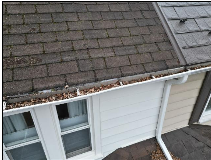
Deteriorating shingles
