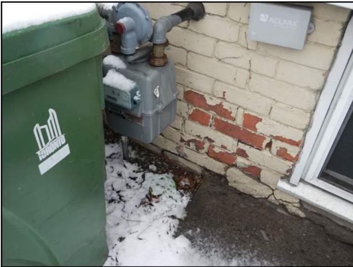
Masonry deterioration: front
