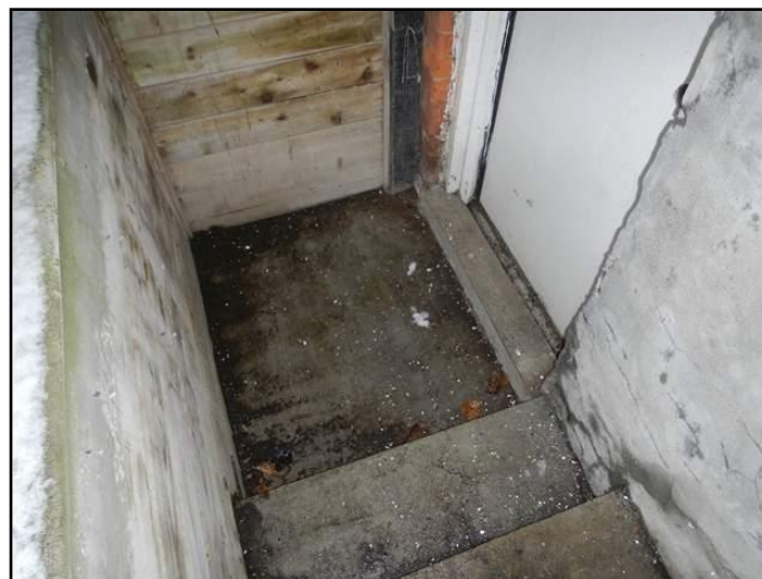
Drain - missing
